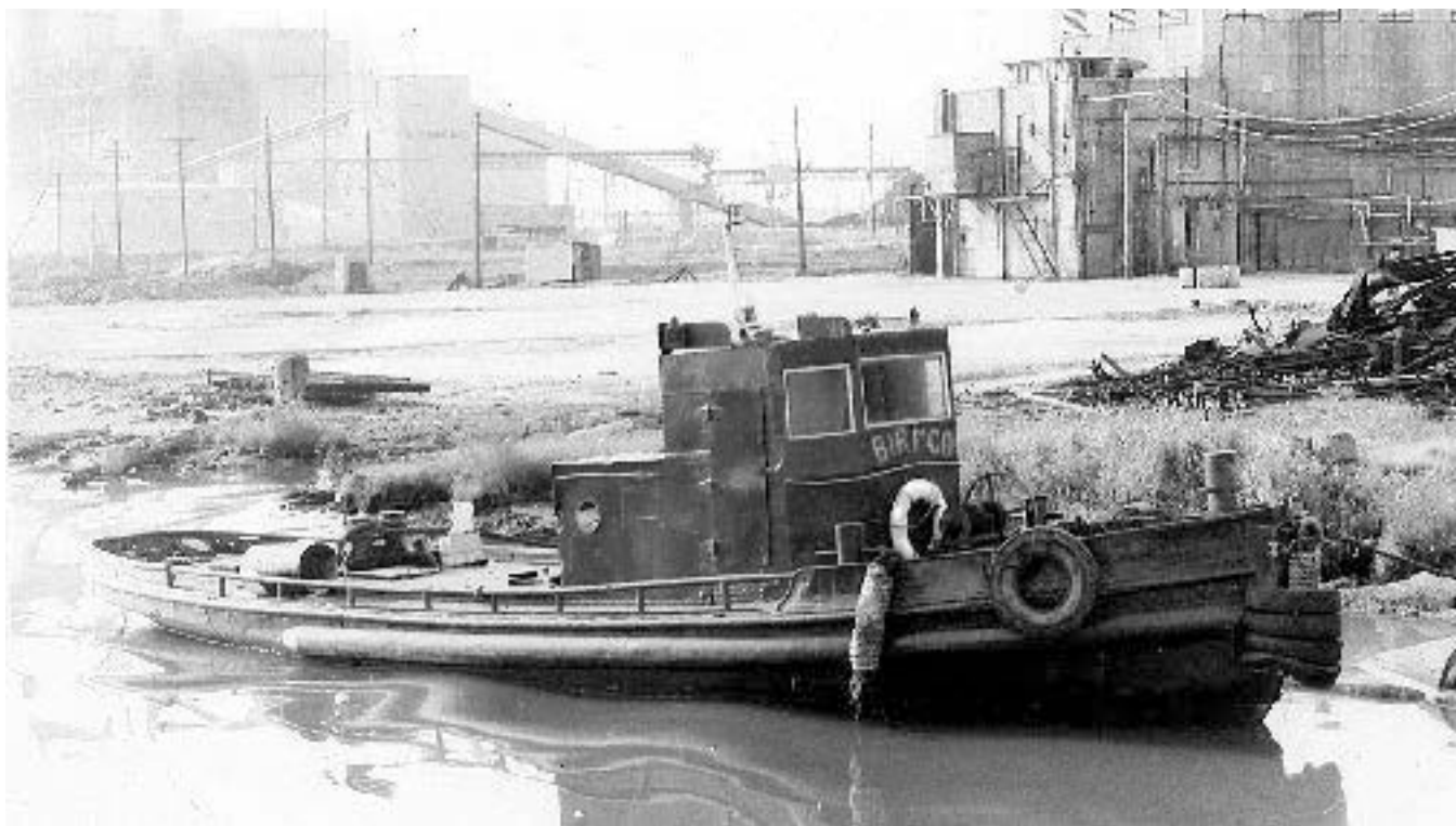
Birmco being repowered c1946 in the Rouge River [DC]
