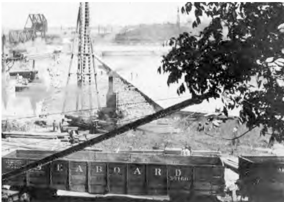
Wet dock slip being dredged and pilings driven at Ashtabula [AM]
