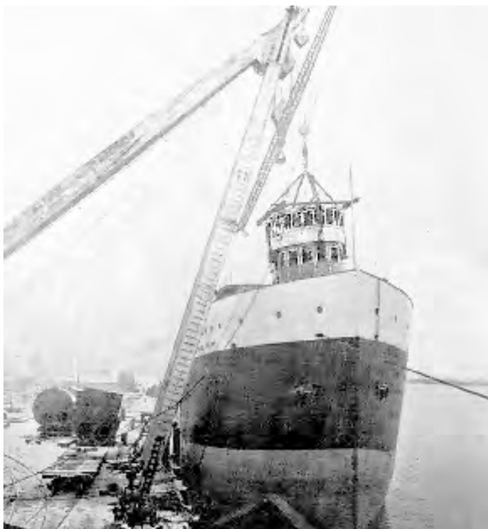
Shear legs placing pilothouse on Jacob T. Kopp - Ecorse yard [GLEW BKLT]
