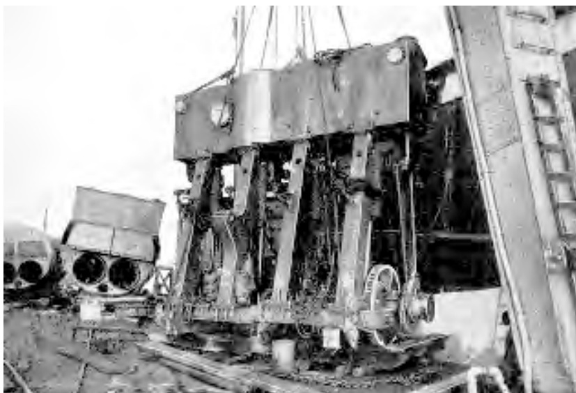
Moll engine and boilers ready for installation at the Ecorse yard 1909 [GLEW BKLT]
